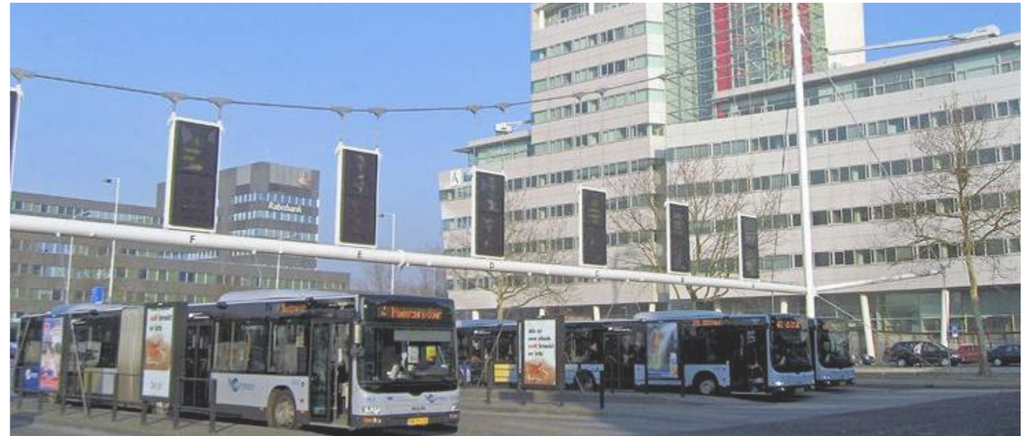
Unsafe and unsufficient busstation
