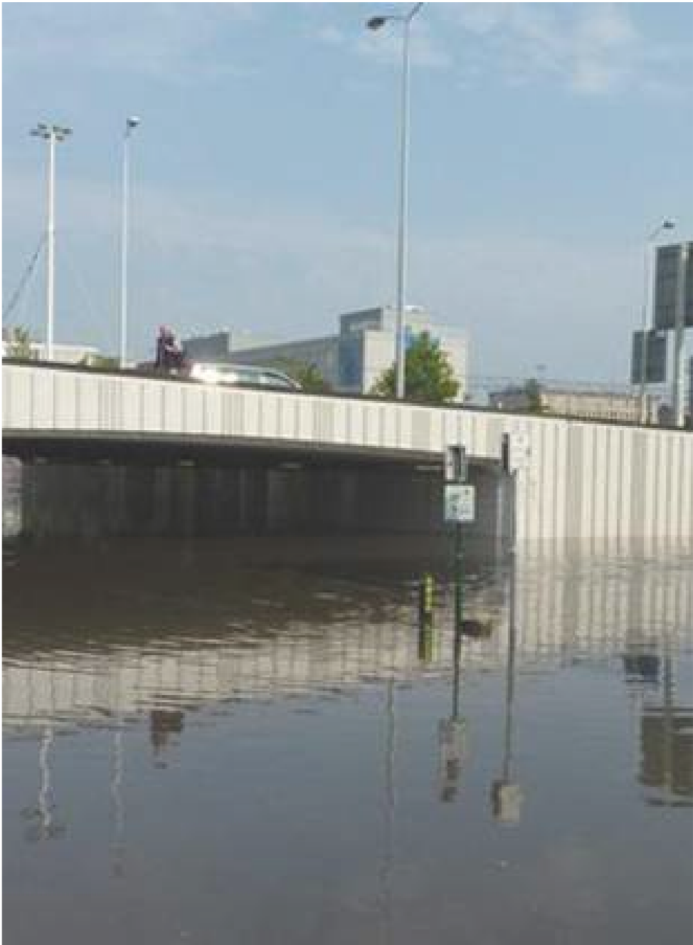
Flooding of tunnels
